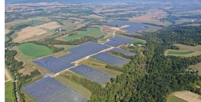
20 MW grid-scale system
